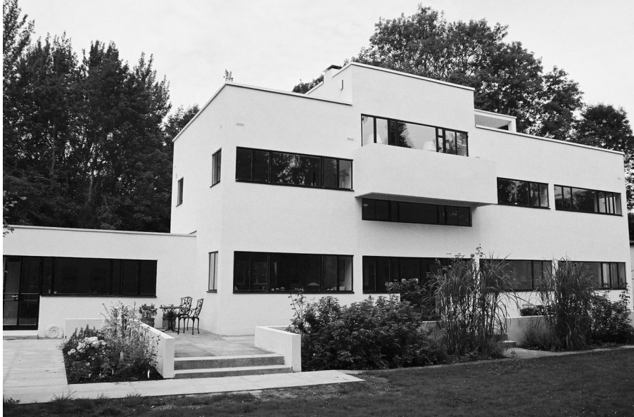
Figure 3 Refurbishment involves both repairs and design. Refurbishment at Willow House, Cambridge (listed Grade II*) included new external insulation, with all windows other than the one under the balcony replaced with double-glazed units and moved out to new positions. 22
