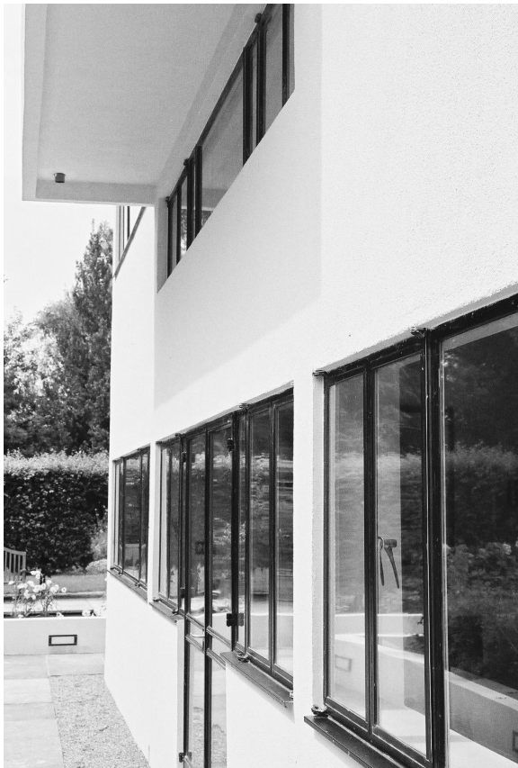
Figure 3 Refurbishment involves both repairs and design. Refurbishment at Willow House, Cambridge (listed Grade II*) included new external insulation, with all windows other than the one under the balcony replaced with double-glazed units and moved out to new positions. 22
